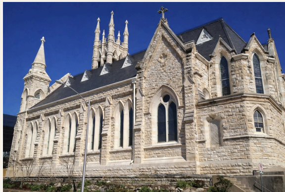
Saint Mary's Cathedral · Austin, Texas · Ash Masonry Masterworks
